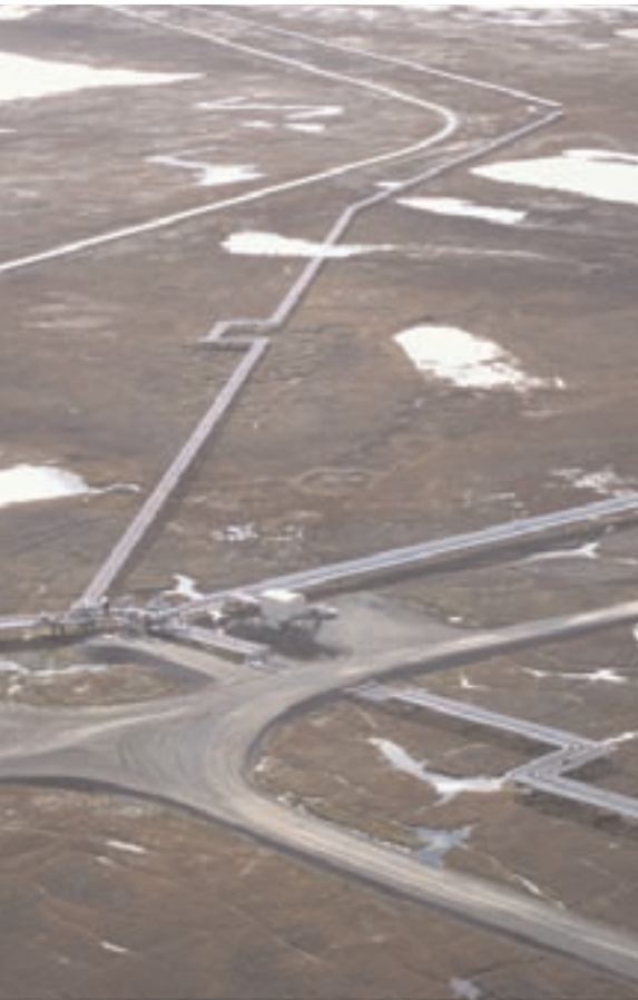
Kuparuk oil field roads, pipelines, and production facilities, September 6, 2001.
