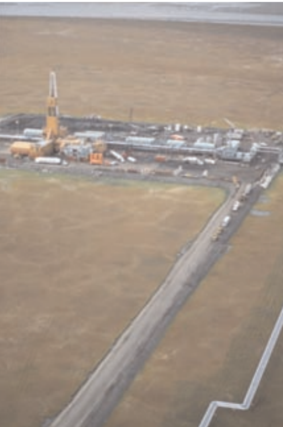
Even the brand-new oil field at Alpine includes miles of permanent gravel roads.
